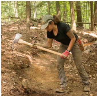
Trail Construction at the Fairgrounds.
